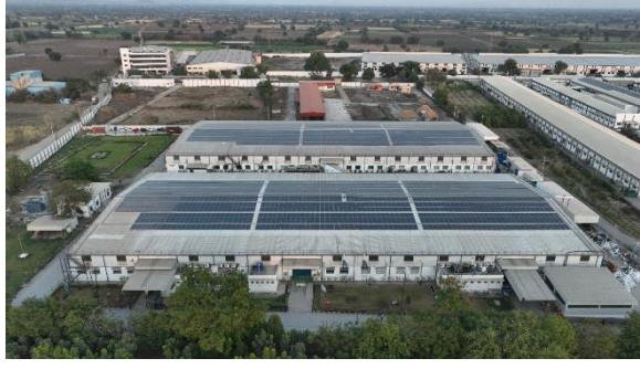
Wiring Harness plant at Shendra, Aurangabad
