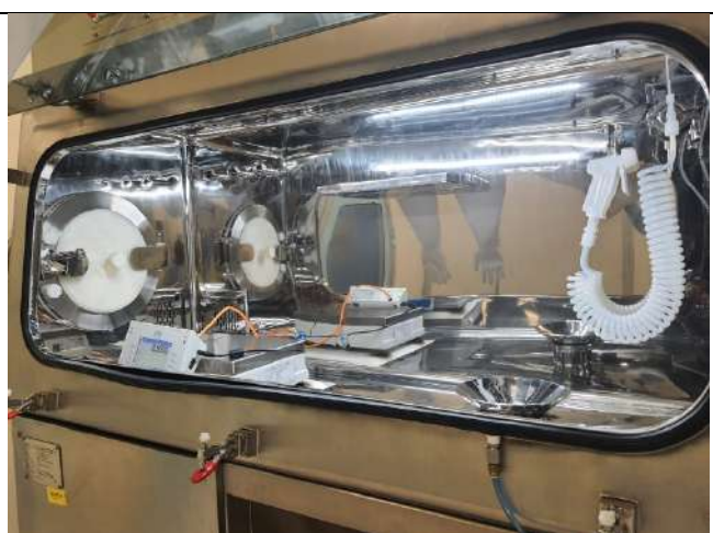
Supplied, installed, commissioned and calibrated sampling isolator
