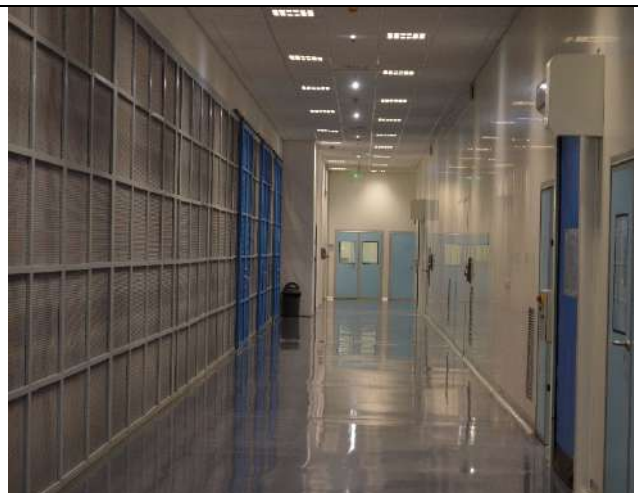
Cleanroom walls, ceiling and view panels installed in a warehouse along with epoxy flooring
