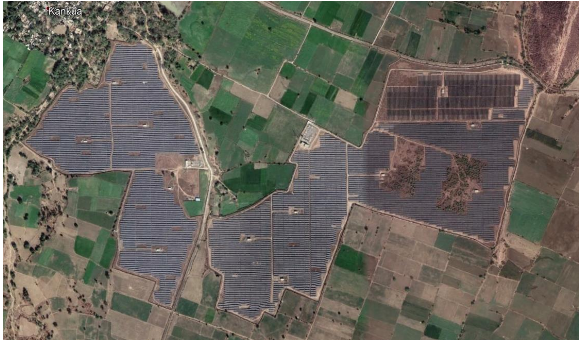
Figure 2-1: Satellite image of 30MW AC plant
