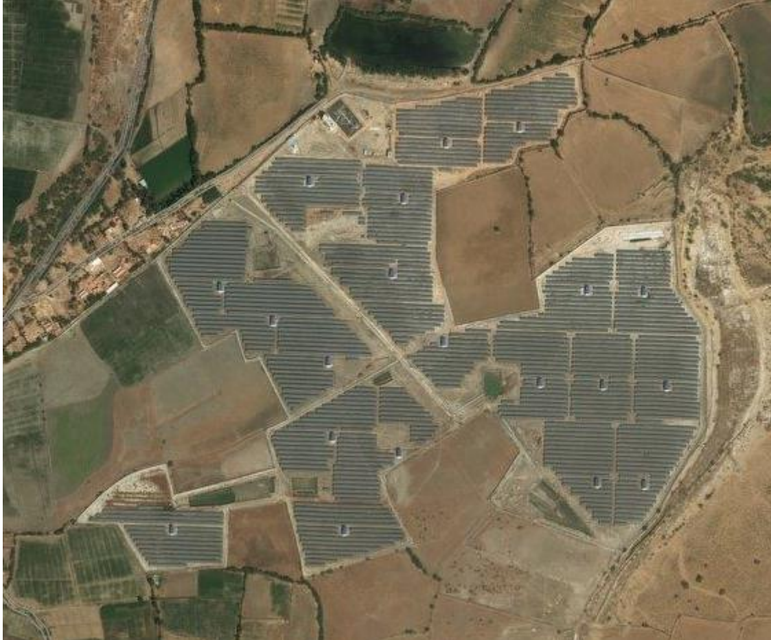
Figure 2-1: Satellite image of 20MW AC plant
