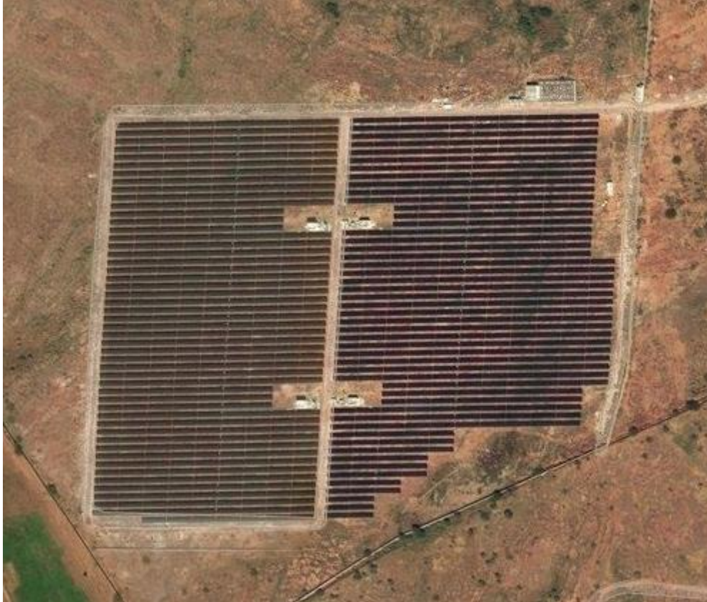
Figure 2-1: Satellite image of 5MW AC plant
