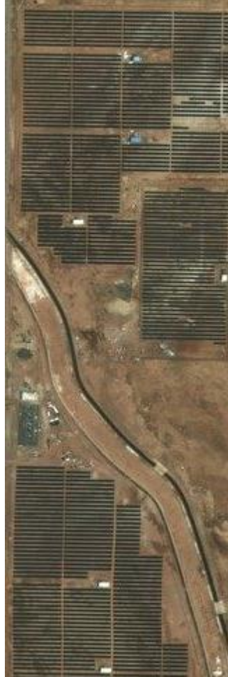
Figure 2-1: Satellite image of 13MW AC plant
